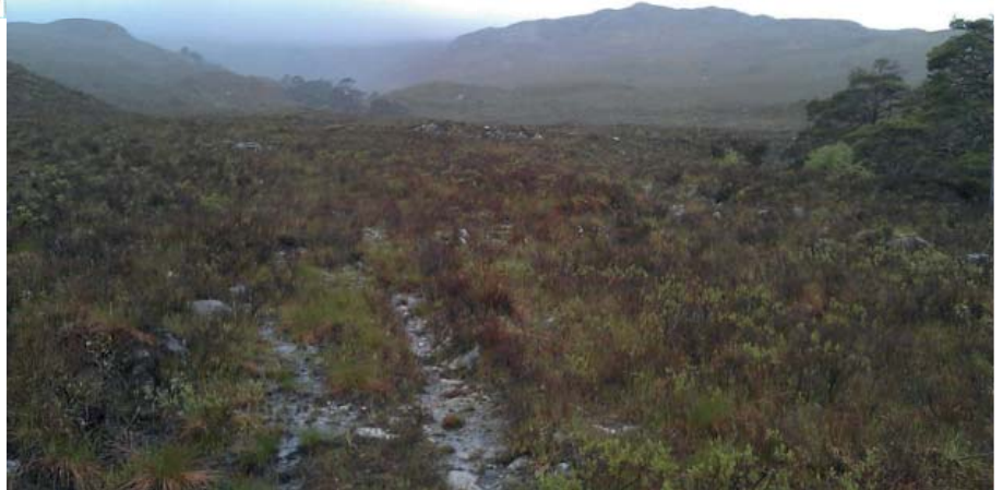
Kinlochewe - The existing Water Treatment Works site prior to the construction of the new works.
