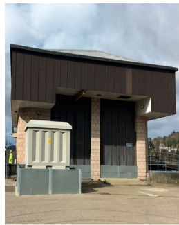
Inchgarth Pumping Station
