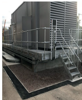
New standby generator platform
